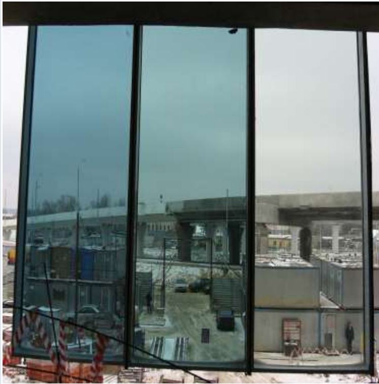
Pyrolithic coatings on body tinted glass
